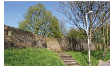
11 Disused pathway into site from Carnoustie Drive
