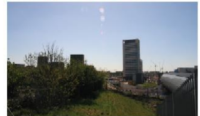
5 View over CTRL Tunnel looking west towards Kings Cross
