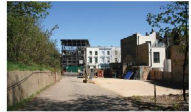
2 Internal access road
