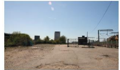
5 Concrete plateau looking west towards Kings Cross
